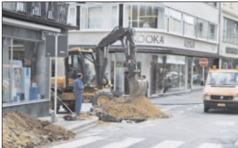
Picture 014 > Bad protected works In such situations, the risk of accidents is very high
